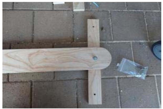
Bolt the Front Steering Rail (#5) to the Main Strut
