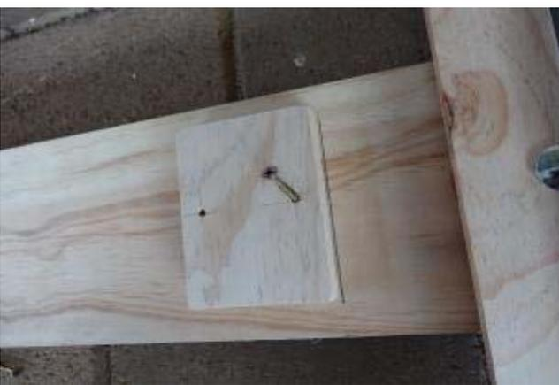
Once happy with the steering blocks position Screw it down with 2 Counter sunk screws
