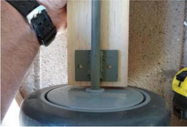
Line up the Rear Axle so it is center and equal gaps are present at each end and Screw Down
